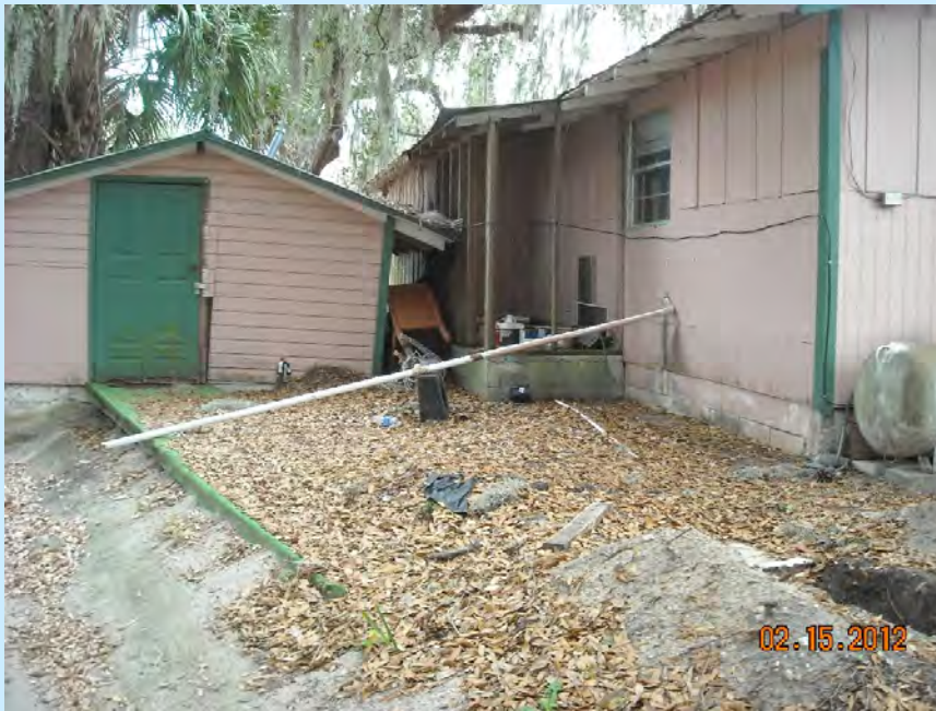
Washing machine discharge
